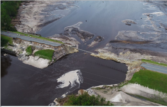
Dam breach at Boiling Springs Lake, NC
